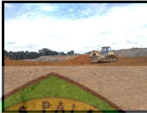
Gambar 4.4 Penebaran Topsoil
